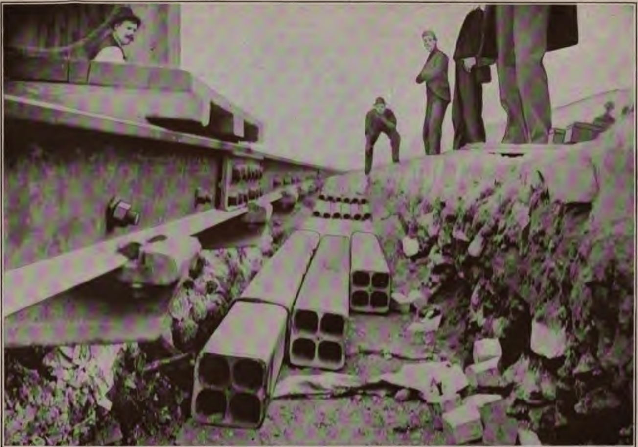
TELEPHONE CONDUITS NEAR STREET RAILWAY TRACK.
